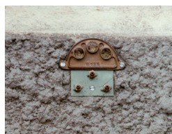
Plaque 3 trous ø 20 Buse longue ø 4
