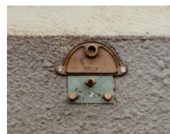
Plaque 1 trou ø 14 Buse courte ø 4
